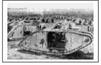
**Tanks** were used for the first time in the First World War. They were developed to cope with the conditions on the Western Front. The first tank was called 'Little Willie' and needed a crew of 3. It had a revolving turret, and its maximum speed was 3mph. It could not cross trenches, however.
